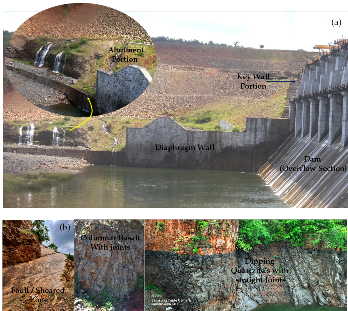
Fig.4 (a) Geology near dam abutment (b) Typical geology observed surrounding dam site
