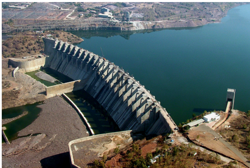
Fig. 16 Panoramic view of Indirasagar Dam
