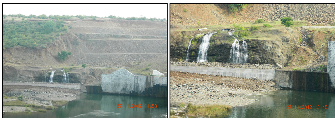
Fig. 1. View of the Spring Discharge on the Right-Hand Side of the Dam
